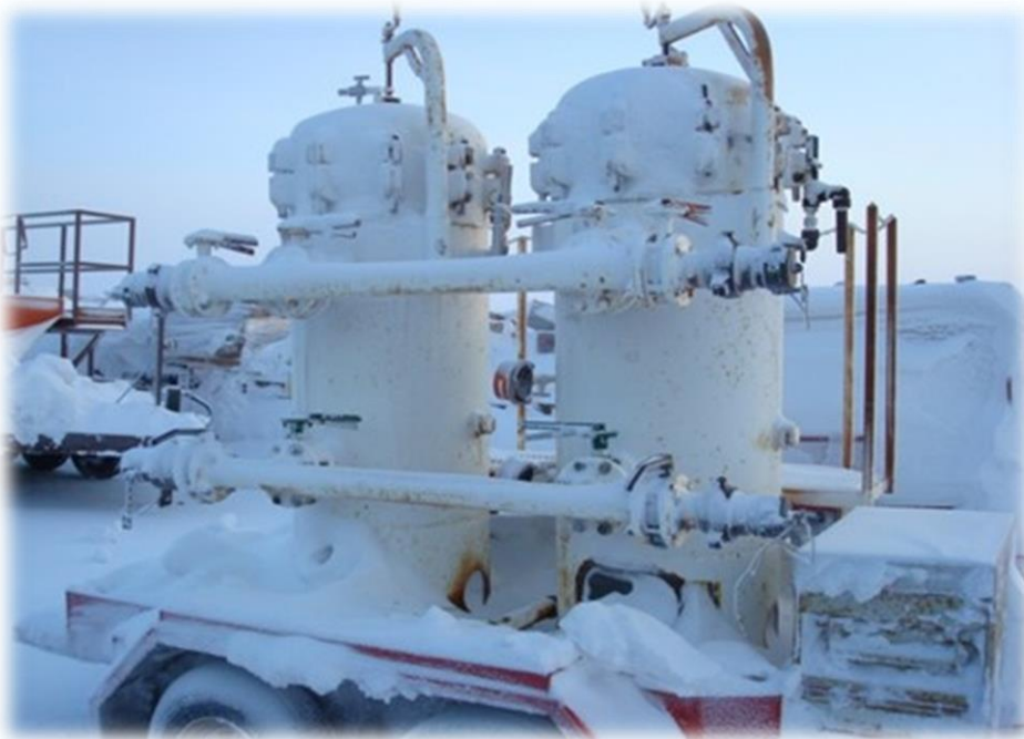
Trailer-mounted dead-end filter pods
