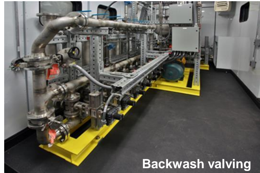
Fully skidded filter system
