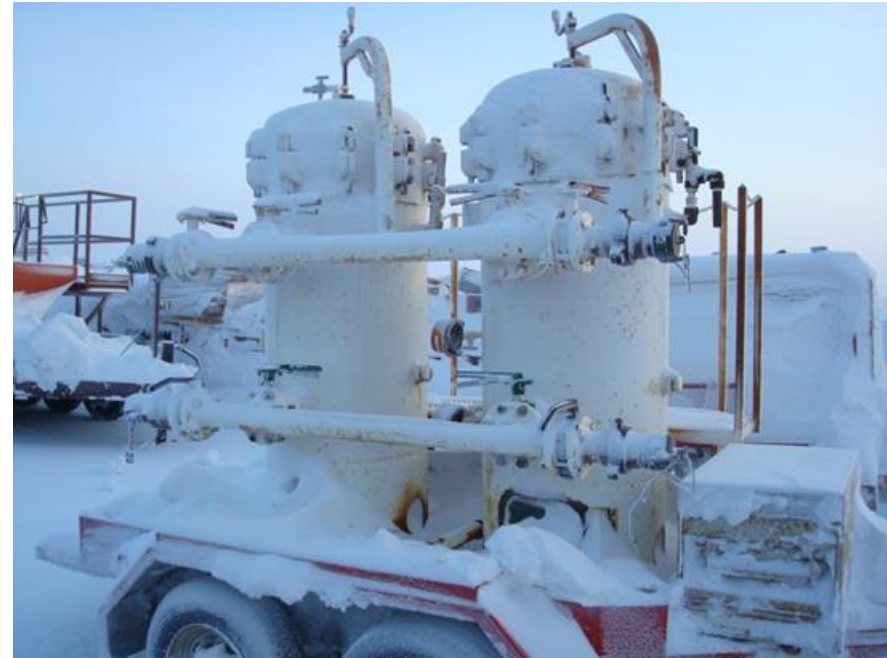
Trailer-mounted filter pods
